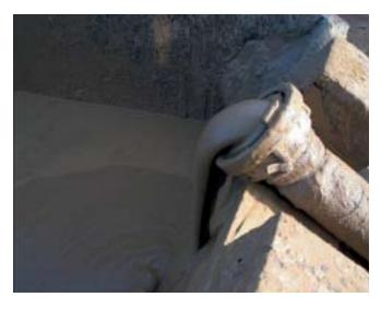
pump which could be used also during pressing. Transporting off was simple as it was possible to pump the drilling material directly into the containers provided.
