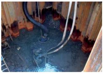
In the event of abrasive and corrosive utilization, stronger wear and tear will take place naturally in certain components. With regards to the above application wear and tear can take place mainly in impeller, suction plate, shaft sleeve, oil ring and mechanical seal. Depending on the working conditions the lifetime of those parts might vary significantly and can be shorter than the legal warranty period.
