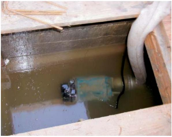
In the event of abrasive and corrosive utilization, stronger wear and tear will take place naturally in certain components. With regards to the above application wear and tear can take place mainly in impeller, suction plate, shaft sleeve, oil ring and mechanical seal. Depending on the working conditions the lifetime of those parts might vary significantly and can be shorter than the legal warranty period.
